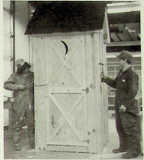
Carpentry's (out house)
