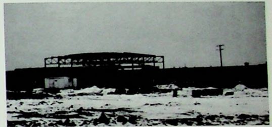
Northwest under construction.
