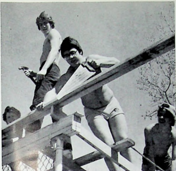
Construction of the new dugout
