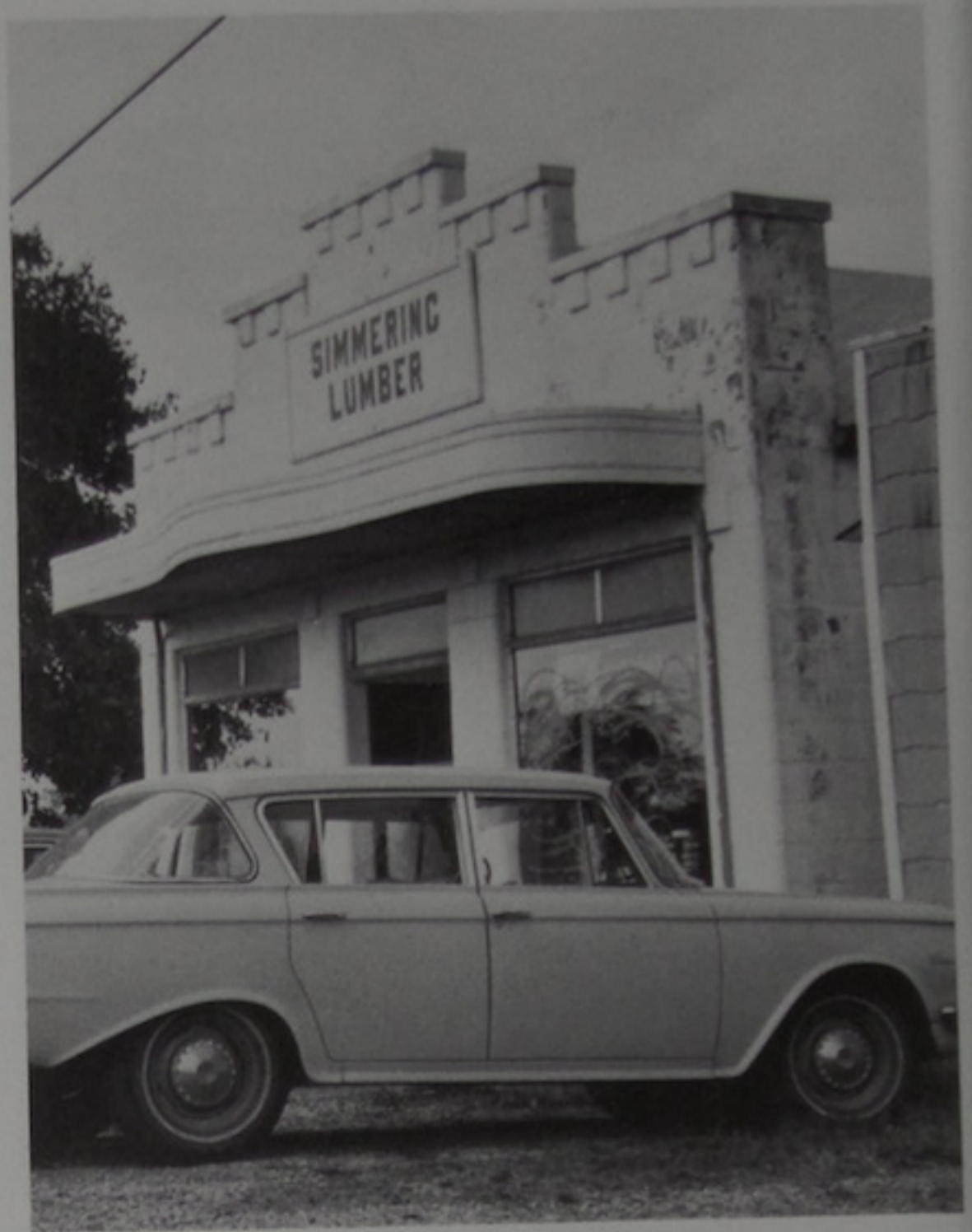
SIMMERING'S LUMBER South Webster, Ohio
